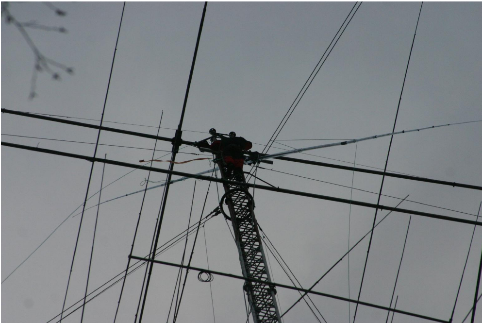
OH7JT up 60 meters installing the upper 80 m dipole 10 hours into the contest. (Pekka OH2HE)
